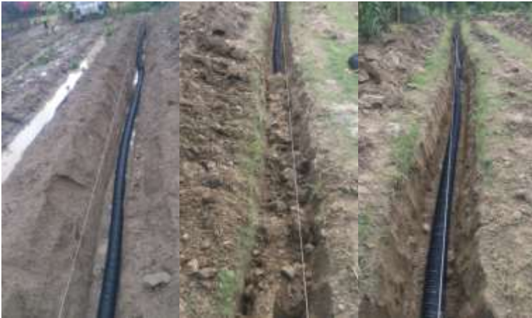
Laying Arched Mesh Pipe
