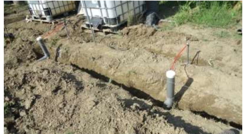
Connect Water Supply System
