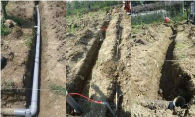
Irrigation and drainage systems connection
