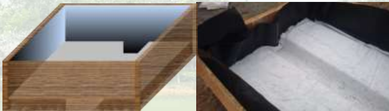
5. Lay textile fabric over mesh pipes
