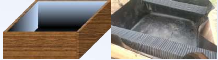
2. Cover water membrane inside the garden edges
