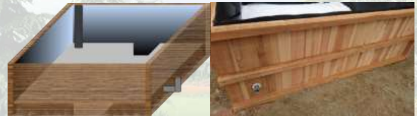
6. Install a mesh drainage pipe vertically as the water inlet and a water overflow pipe
